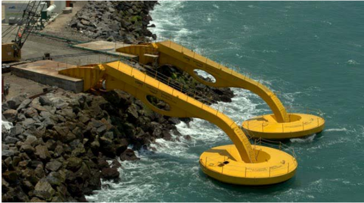
Buoy vertical movement
